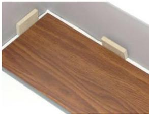
3. The end joints of the planks in the first row are assembled by inserting the tongue side into the groove side of the previous plank at a **low angle**. Gradually lower the plank down flat until the end joint closes, insuring that the planks are perfectly aligned. Install remaining full planks in the first row.
