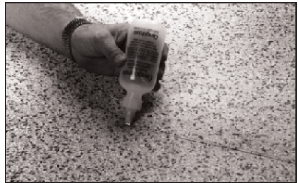
Fig. 8. Hold applicator bottle perpendicular to seam cut.
