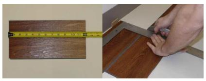
5. The remaining scrap piece cut from the last plank in the first row may serve as the first plank in the second row provided it is at least 12" (30.4 cm) long. Always stagger end joints from row to row a minimum of 12" (30.4 cm).
