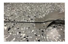
Remove the excess bead from one direction before working the bead from the opposite direction.
