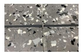
Angle cut or router your bead at the junctions to make it easier to weld in the opposite direction.
