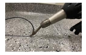
Beginners may find it easier to work with a lower heat. However, with experience, welding will be faster with a higher heat. A lower heat is for correcting mistakes or welding in awkward places. A good weld is achieved when a small amount of melted bead overflows along the edges of the groove.
