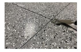
After the weld has cooled, shave off the excess bead with a spatula and height guide. If the bead is shaved before it has cooled, it will shrink below the surface of the flooring. Keep the spatula sharp by periodic honing with a fine sharpening stone.
