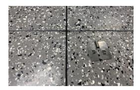
After welding and trimming all the seams in one direction, repeat the router procedure, welding, and trimming procedures on all seams running in the opposite direction.
