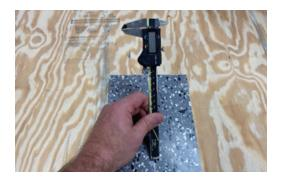
Check the depth of your router cut with a depth gauge and make an adjustment to remove .060". Roughly ½ the thickness of the tile.
