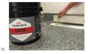
Continue to form the tile to complete your run of straight pieces. Let them cool, then apply the correct adhesive to all areas where the flash cove tile is positioned. Continue to tape the pieces together to hold tight seam.
