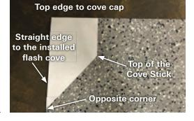
Cut out the piece and warm up the piece with a heat gun and install the piece. Adjustments are not uncommon.
