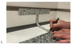
Using your Tile - T, push the flat edge under the cove cap following the radius until you meet the tile edge.
