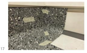
Warm up the corner piece, bending and adjusting the fit until the tile is in place properly. Tape the seams until the tile is cooled.
