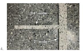
Take one tile and create a Tile - T this is used to measure from the top of the cove cap to the edge of the installed tile.
