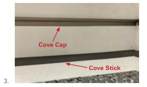
Install Cove Cap and Cove Stick, by using contact adhesive and 1 1/2" masking tape, staples or brads will work to secure. Let the cove cap and cove stick dry over night.
