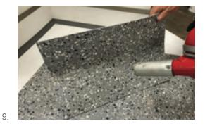
With your heat gun, warm the tile where the cove stick and the tile will meet until it becomes flexible. Keep the heat moving across the piece.
