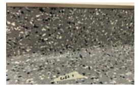
Top edge is 1/8" wider for overlap Notch the top of the tile for the height of cove cap corner Hand cut edges Factory edge
