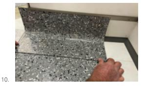
Insert the warmed tile under the cove cap and slowly move the tile in place so the bottom edge slides next to and flush to the installed floor.
