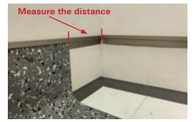
Measure the distance from the installed flash coved tile to the inside corner.
