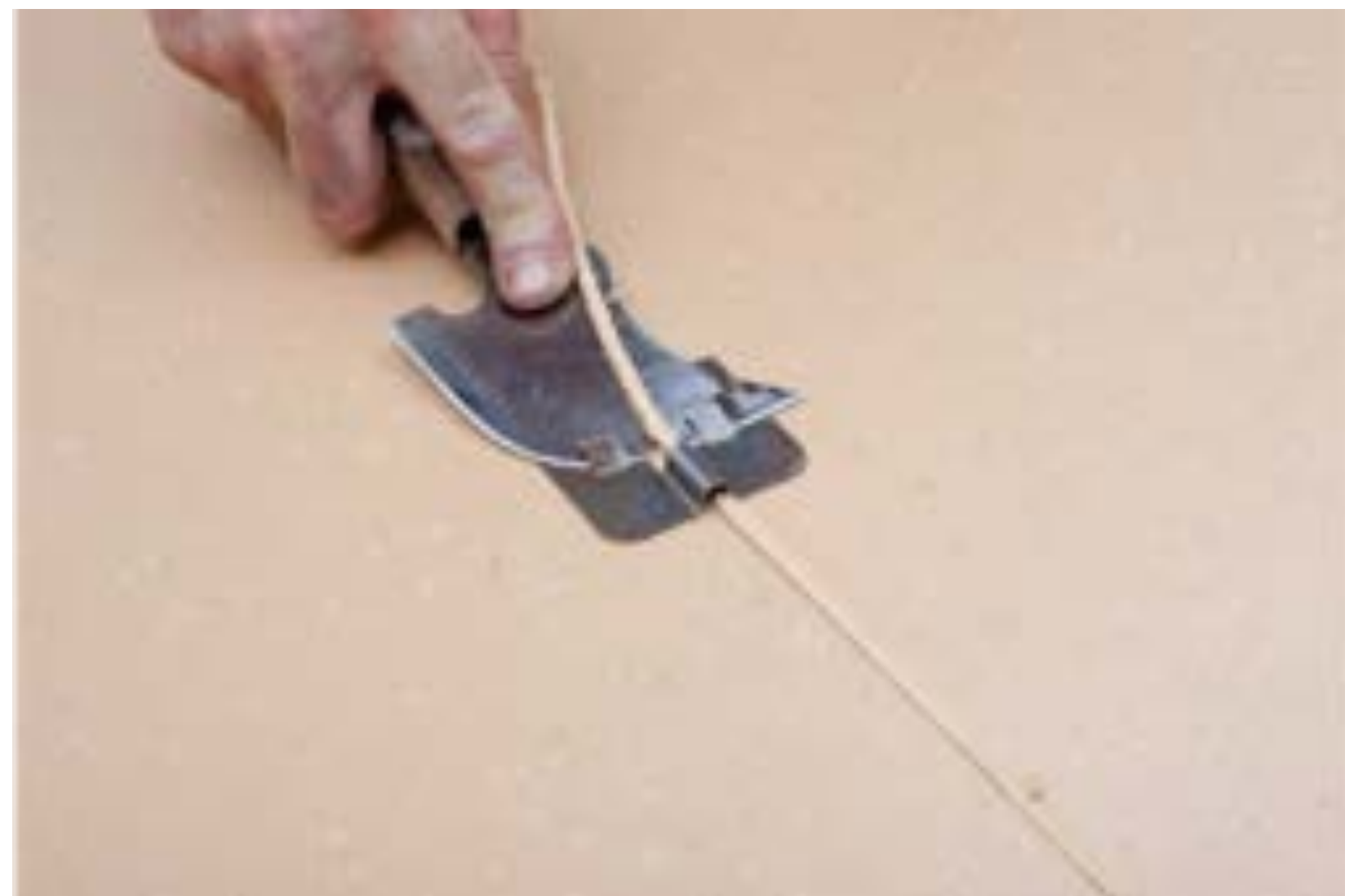
Shaving of weld
