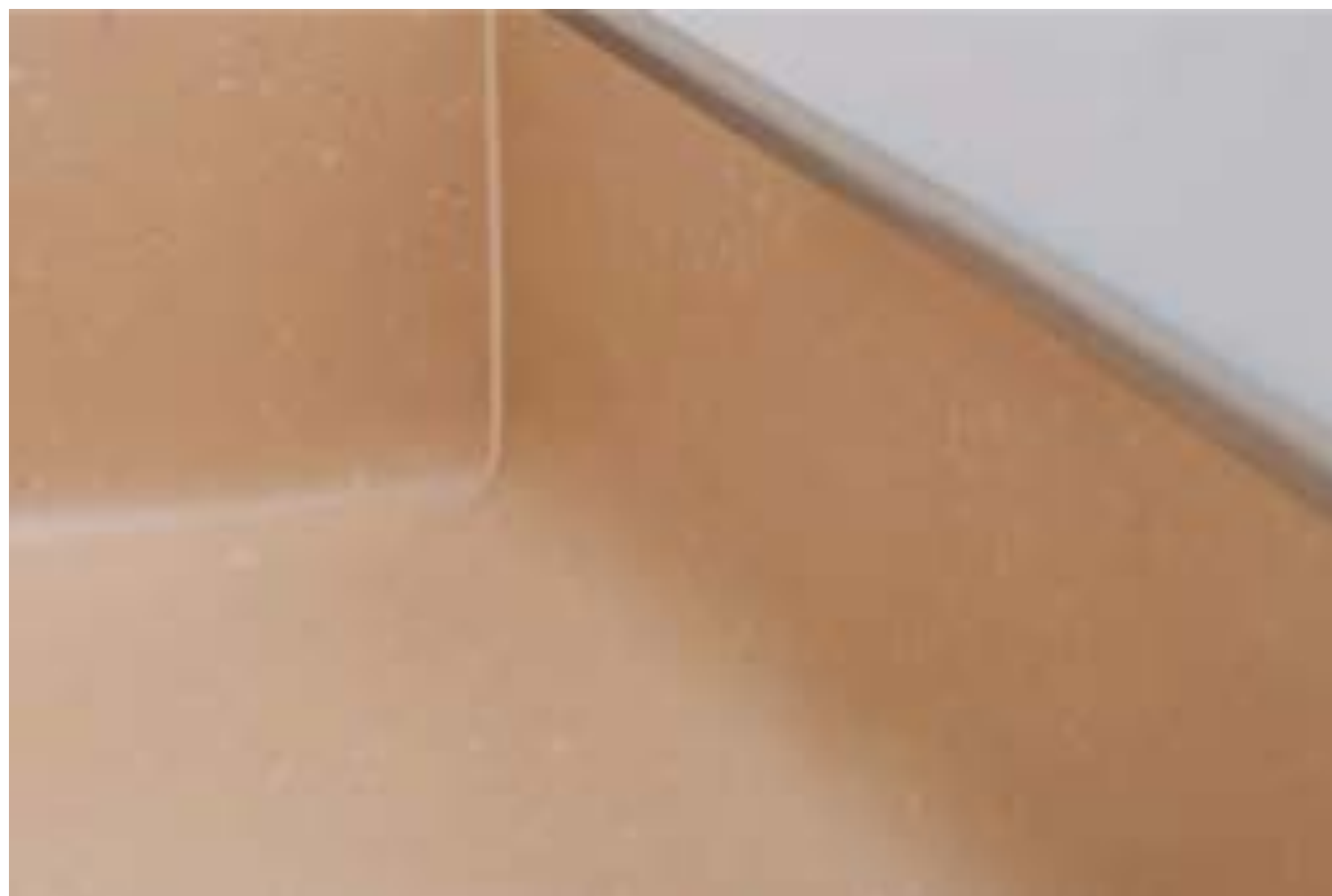
Finish inside weld
