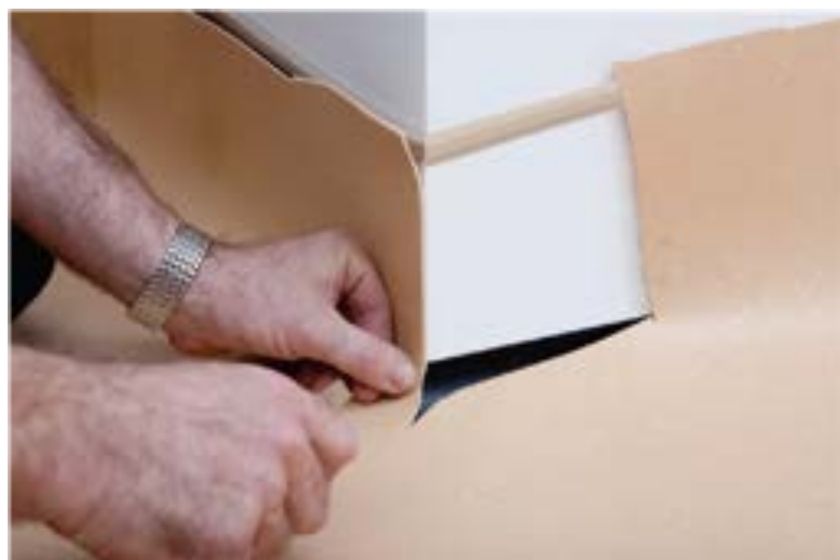
Cut and fit sheet
