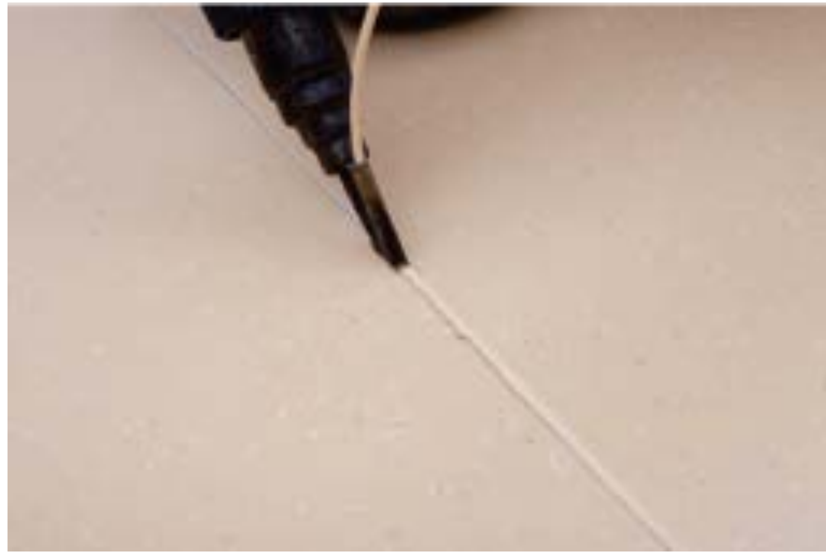
Welding of groove
