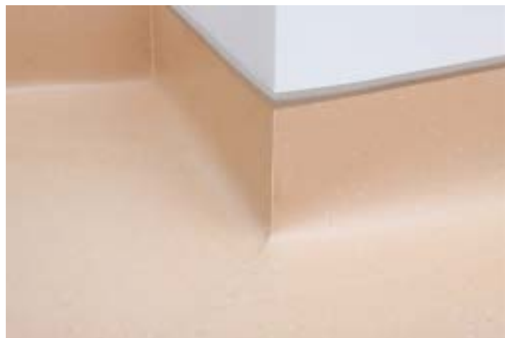
Final look of internal and external corners
