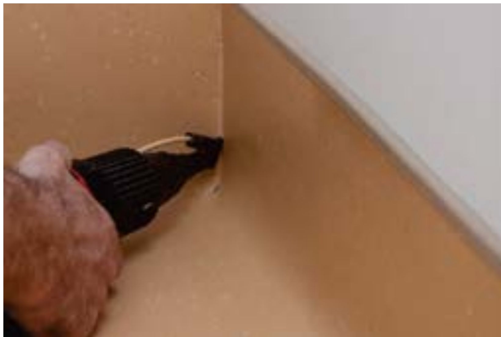
Weld in place
