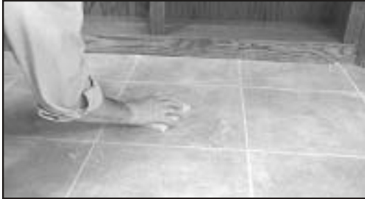
Fig. 17 - Use a 3M white, nylon pad to loosen grout residue.
