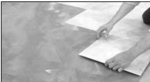
Fig. 12 - Install ungrouted floors following a stair-step pattern.
