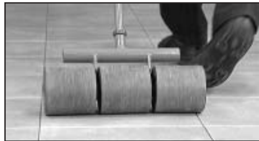
Fig. 13 - Roll the floor within one hour after setting tiles.
