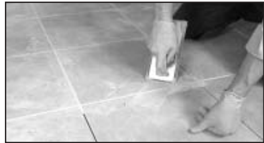
Fig. 15 - Pack the grout into the joints.
