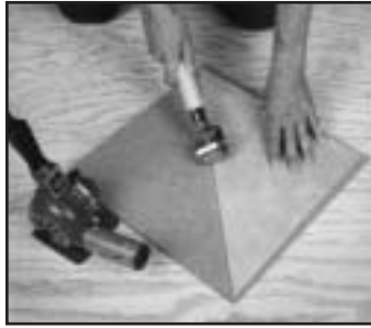
Fig. 14 - Roll the cut edge to form a slight radius.
