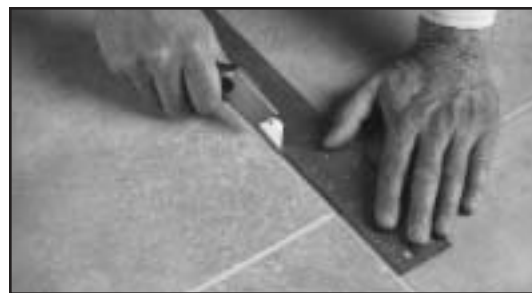
Fig. 18 - Cut along the center of the grout line after heating it.
