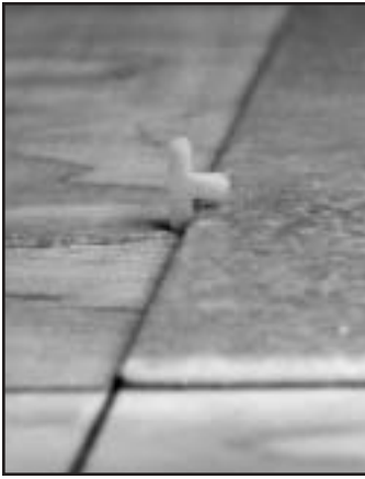
Fig. 10 - Use spacers with one leg removed.
